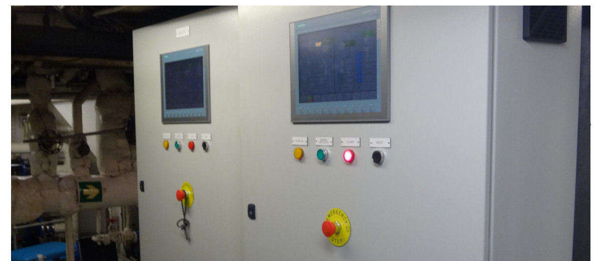
Figure 9: New pre-assembled panels.
