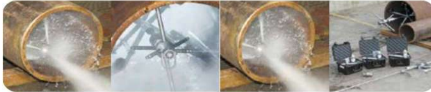
RETRO JETTING DEBRIS PIPE CLEANING PROCESS
