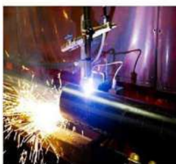
PIPE MACHINE WELDING
