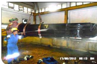
HEAT EXCHANGER HIGH PRESSURE WASH
