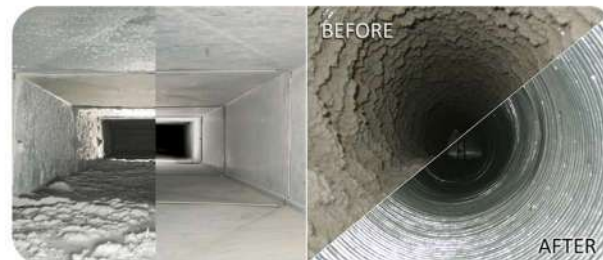
Air Ducting Clean Before & After
