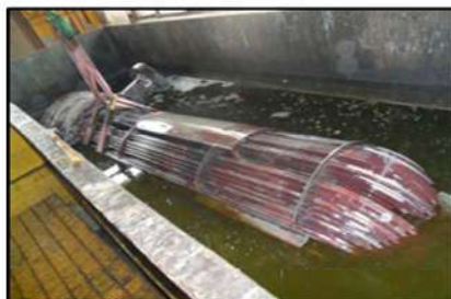
HEAT EXCHANGER CHEMICAL CLEANING WASH
