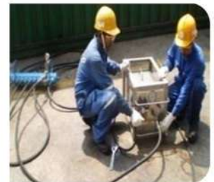
PRESSURE TESTING PROCESS
