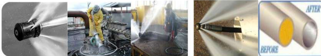
WATER JETTING PROCESS AND PIPELINE JETTING PROCESS
