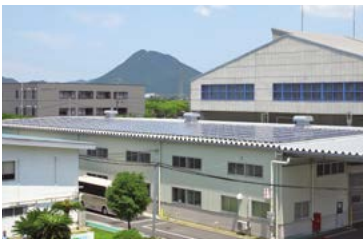
Photovoltaic power generation
