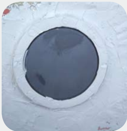
New anode installed
