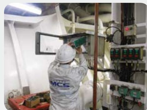
Inspection & repair on MGPS panel
