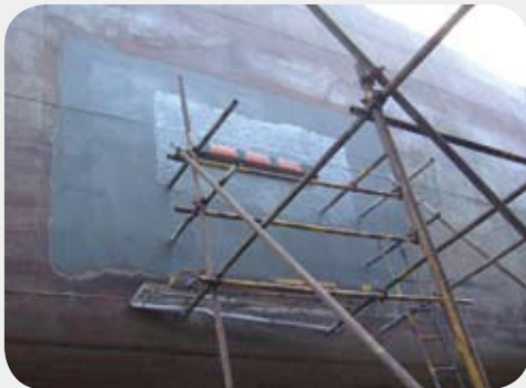
ICCP Linear anode renewal work
