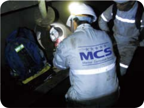
Anode renewal work in the tank
