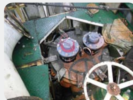
MGPS anodes on strainer's lid
