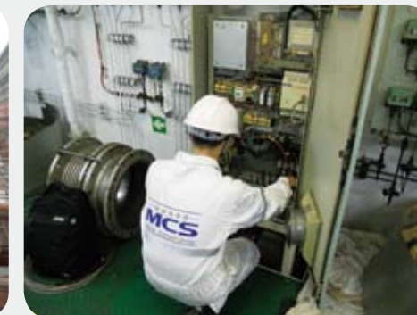
Fault finding on the ICCP power unit
