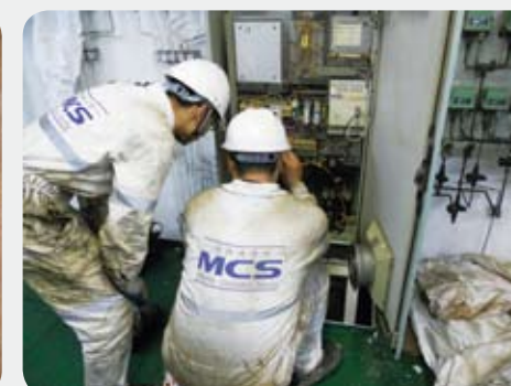
ICCP system inspections on the control panel
