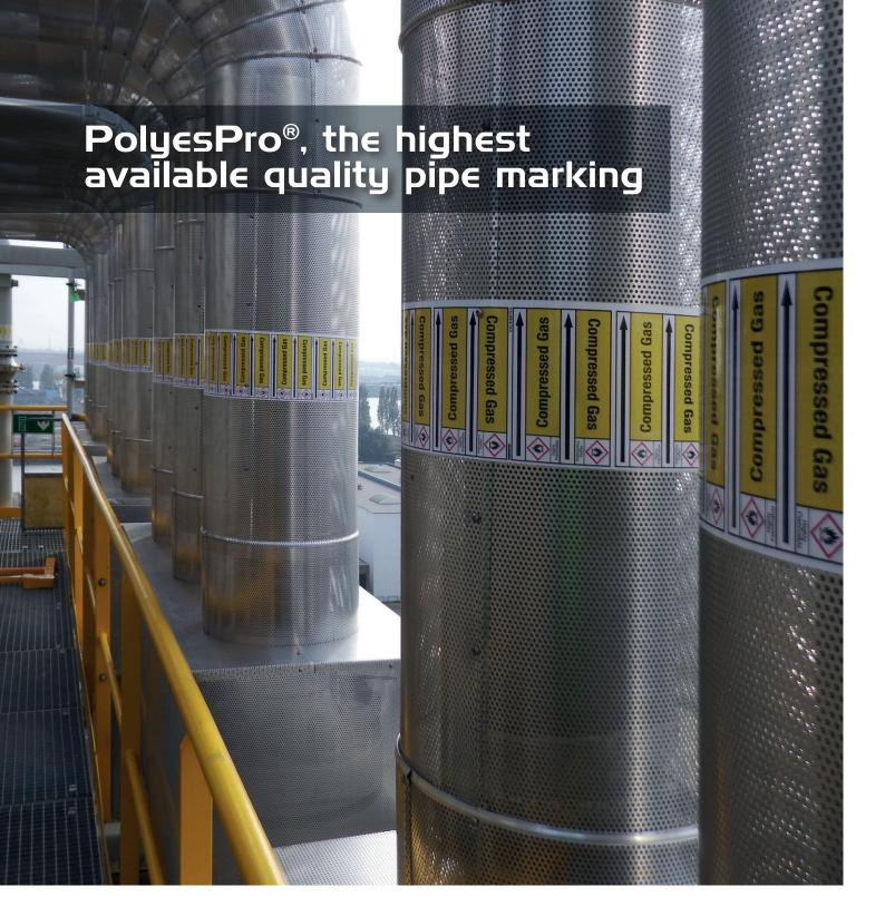
We are supplier of the specially developed PolyesPro® pipe markings. This product has a better temperature resistance, therefore a longer service life and improved colourfastness. The tape comes with all the usual 3M™ guarantees. PolyesPro® pipeline markings are made out of two layers; a PVC free polyester base material with the image, finished with a protective laminate. As a result, the material is suitable for insulated pipes, painted pipes and stainless steel pipes.
