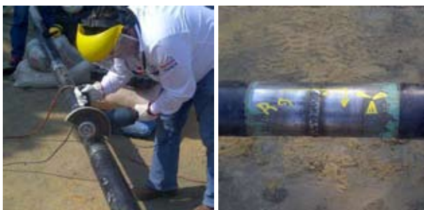
On working using a grinding machine the result is uneven and incomplete cleaning of the material, hardly any surface roughness
