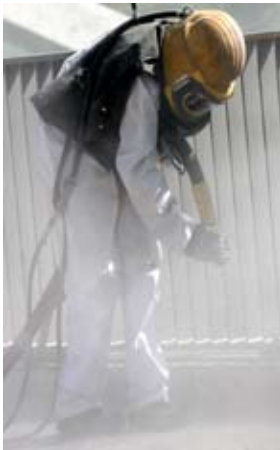
Conventional grit blasting
