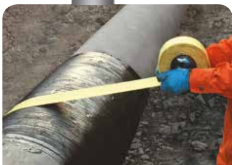
PIPE REPAIR & REINFORCEMENT
