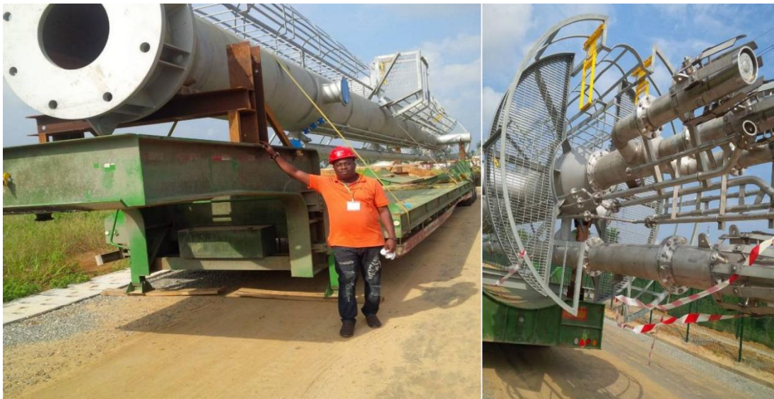
OJMATS: 2015, Heavy weight lift of Burner boom
