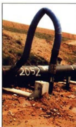
▲ REPAIR OF HOLED PIPE FOR WATER SUPPLY AND DRAINAGE PIPELINES
