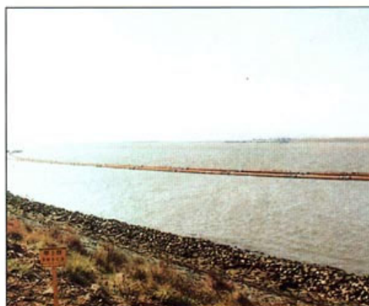
▲ TRANSPORTING LINES FOR SAND
