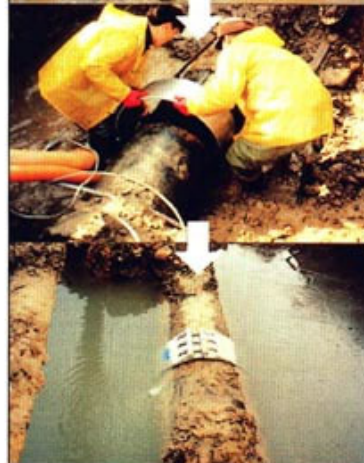
▲ EMERGENCY REPAIR SITE FOR UNDERGROUND WATER SUPPLY LINE
