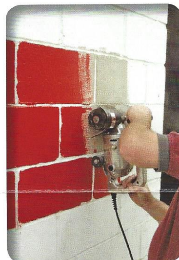
Coating Paint Removal
