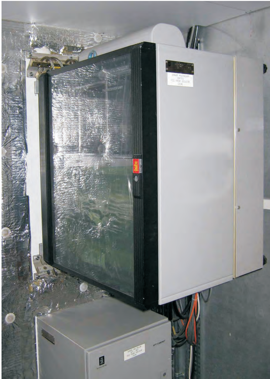
Figure 24 Installation of the Transceiver Unit on “HMS Endurance”
