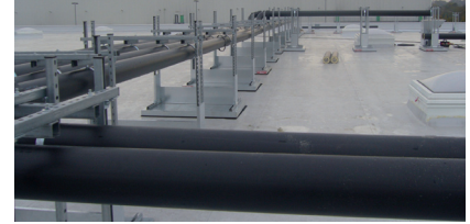
COOL-FIT ABS Plus pipe installation on the distribution center roof.
