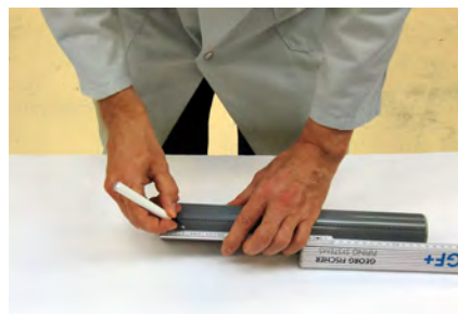
Marking the joining length
