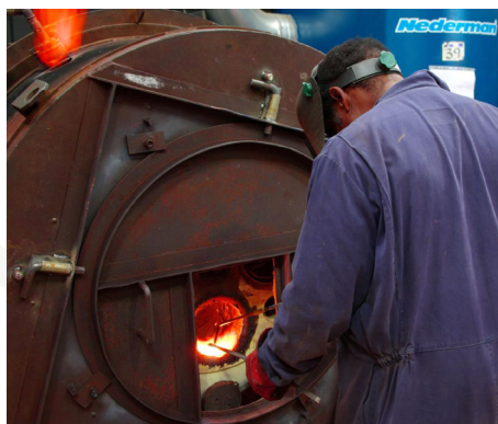
The cylinder cover during the welding process
