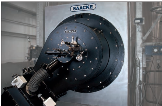
The DDZ-M in operation, here on a 12 t/h boiler
