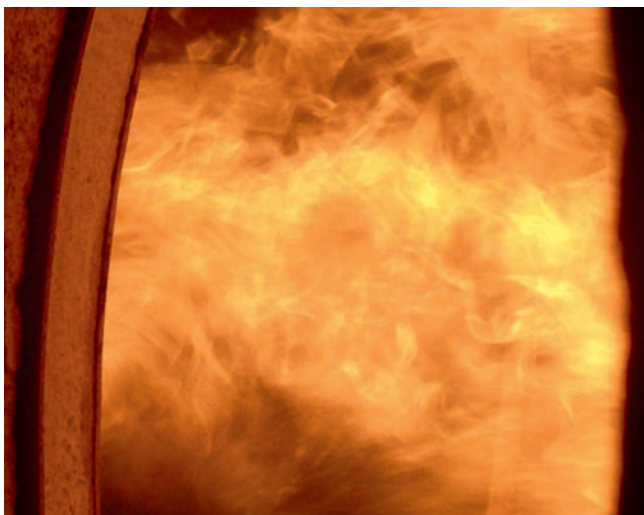
Typical DDZ-M heavy fuel oil flame
