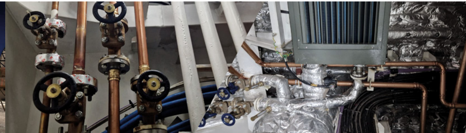
Replacement of 150 m hot water pipe system on LNG carrier. Location: Klaipeda, Lithuania.
