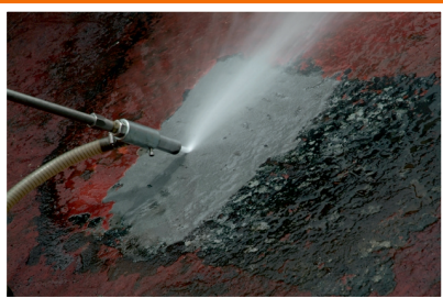
Surface - Sand Blasting
