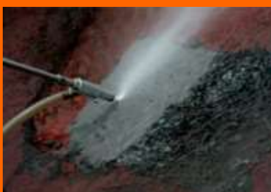
Surface – Sand blasting
