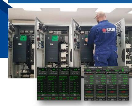
**SELMA SEES** Ship Energy Efficiency System is a reliable method/application in order to reduce a vessel's fuel consumption by optimizing its power balance and in parallel by adapting the operation of the Cooling Sea Water Pumps and E/R Fans to the actual power requirements.
