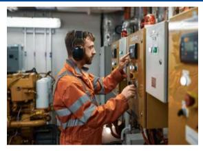
**SELMA Engine Room Personnel Alarm System** (**Dead Man Alarm**) is used when the Engineer on duty enters the Engine Room where the system must be set in operation from Remote On/Off Stations and the timer counter must be reset from remote stations in order to ensure acknowledgement that the Engineer on duty has entered E/R. After exiting the E/R the Engineer must put turn off the system from On/Off remote stations.
