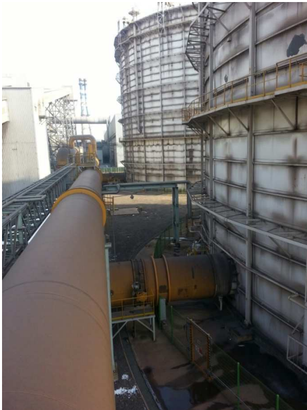
HYUNDAI STEEL Gas Holder Main Line 2700A Fluid : LDG
