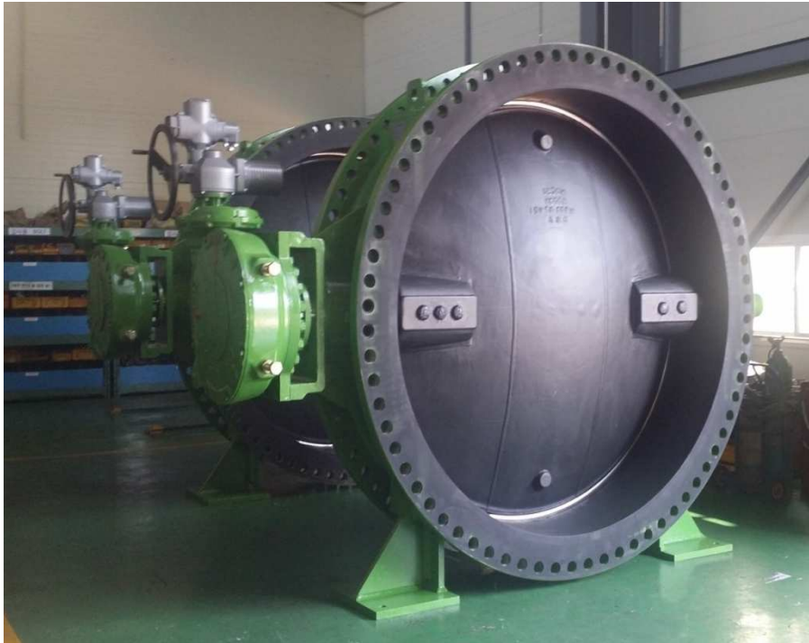
Motor Operated Butterfly Valve Size : 2850A Project : Malaysia Tenaga Nasional Berhad 3A Fast Track Service : CCW H/E B Outlet Fluid : Sea Water
