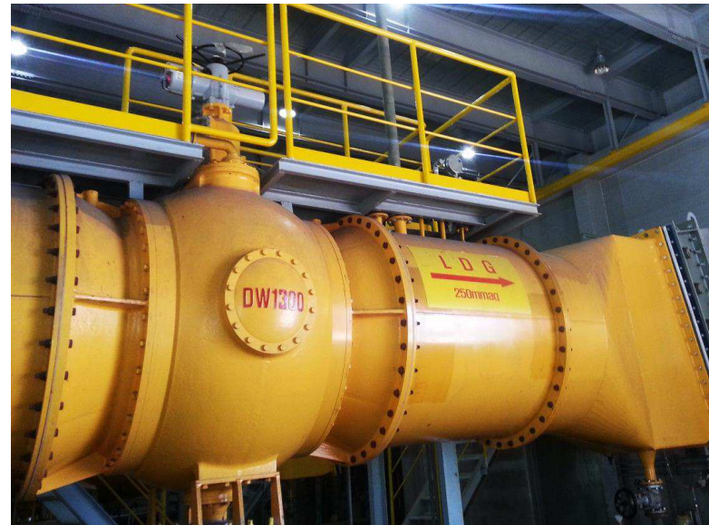
POSCO KWANGYANG Gas Holder Main Line 1300A / LDG Booster COG inlet Waterseal Valve Fluid : LDG
