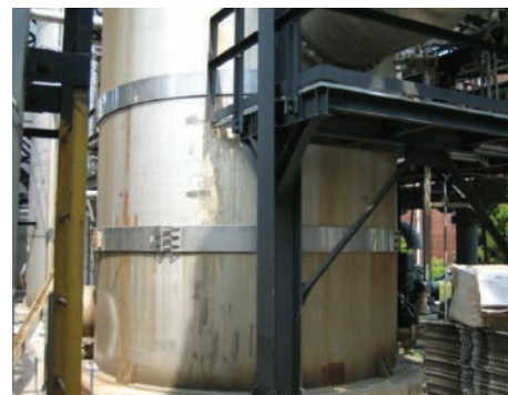
MJFL Viton 3,615mm. chemical storage tank. for protection of weld. Korea
