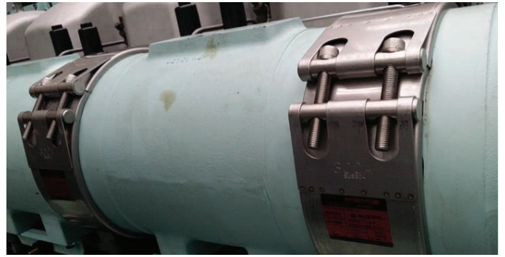
MJS NBR + strip insert 335mm, etc. medium speed propulsion engines & marine genset. Korea
