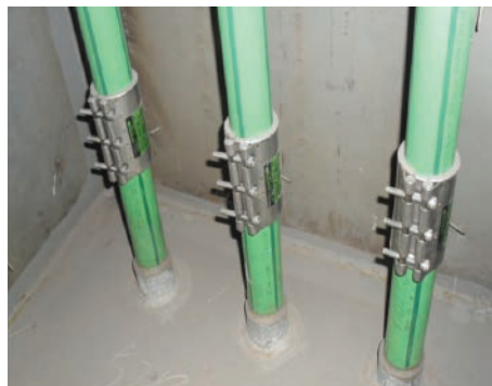
MJGL EPDM 40A. water supply line. PPR pipe. Korea
