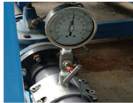
MJD-A EPDM 100mm. pressure gauge installed on PVC pipe. water supply line at power plant. Thailand
