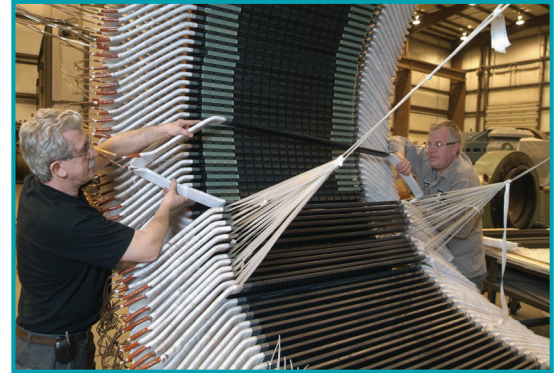
IPS technicians perform an IntegraCoil B-stage hard coil rewind on a high-voltage stator too large to VPI
