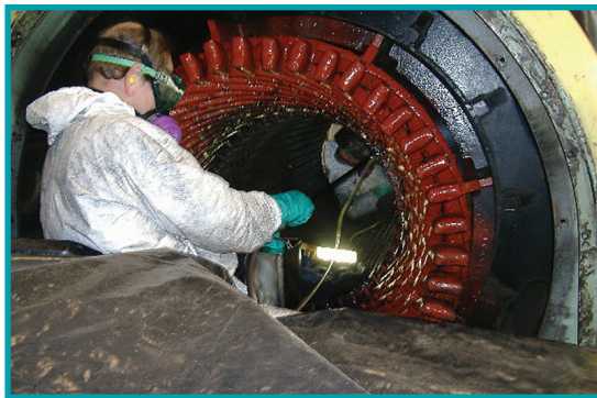
6 MW, 4160 V, 3600 RPM — generator stator cleaning
