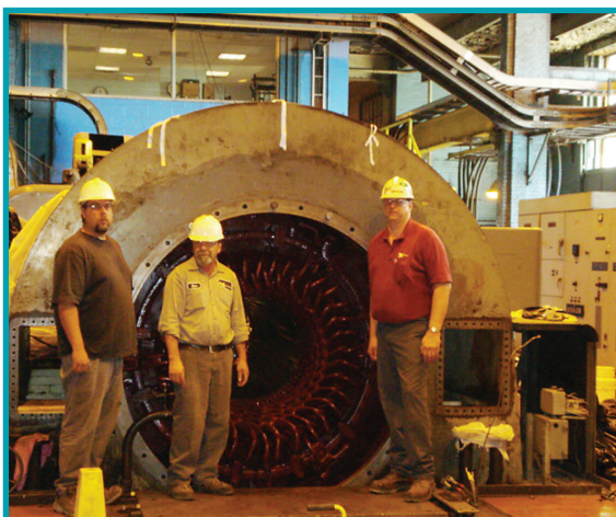
Before and after an on-site rewind of a 22 MW, 13.8 kV, 3600 RPM generator with IntegraCoil™ B-stage hard coils
