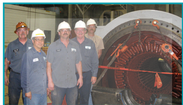
On-site inspection and recondition of 44 MW generator
