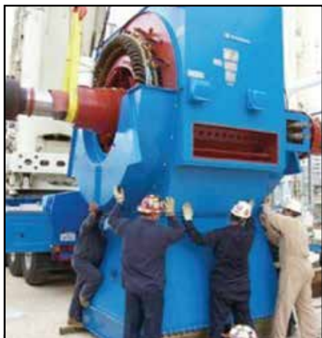
Commissioning of a 21,000 HP main air compressor motor in the Southeast.
