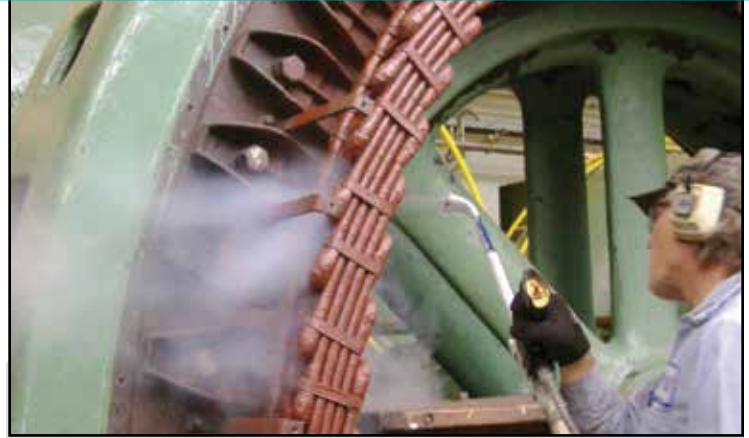
Cryogenic cleaning—one of the many IPS Big Iron services designed to deliver reliability.
