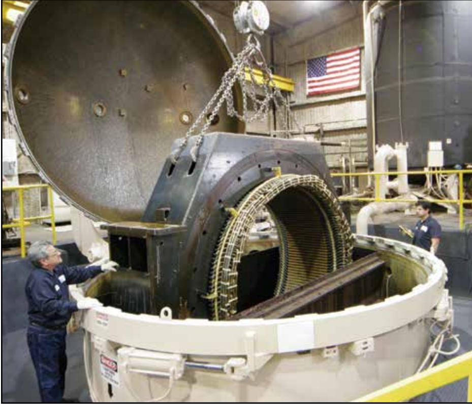
Technicians lower a MegaSeal™ high-voltage rewind into the 14' diameter VPI tank—the biggest in a U.S. service center.
