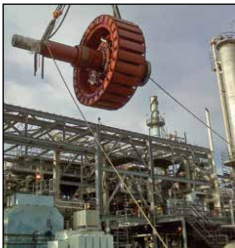
Installation of 7,000 HP synchronous rotor at a west coast refinery.
