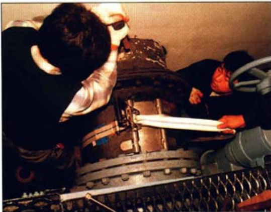
▲ VIEW OF INSTALLING A REPAIR CLAMP(RC-L) ON 500mm DIAMETER PIPE WITH SPECIAL BELT
